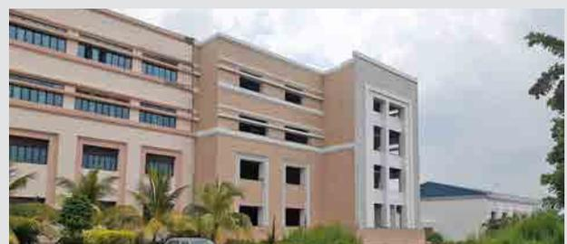
SMS Extension: Structure completed, finishing work such as painting, Aluminum work, false ceiling work, Sanitary work, HVAC & electrical work is in progress. About 71.70% of building work completed.
