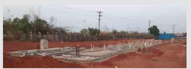
**STP:** Collection tank, intermediate and clear water tank completed. The lab cum control room structure work completed and finishing work, plumbing work, machine installation work and electrical works in Progress. About 67% of STP work completed.
