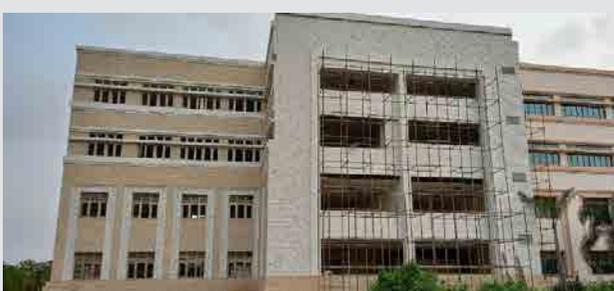
SBS Extension: Structure completed, False ceiling, expansion joint, aluminum work, Sanitary work, electrical work, HVAC work is in progress s. About 78.60% of building work completed.
