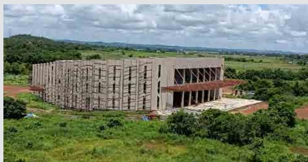
Auditorium: External Cladding, terrace screed concreting, flooring and water proofing work, HVAC chiller foundation & pump room plinth beam work in progress. About 55.69% of building work completed
