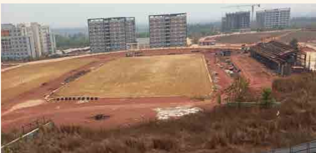
Football, athletic track and javelin ground: About 50% work completed.
