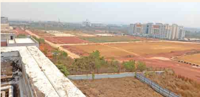
Hockey ground: About 85% of work completed
