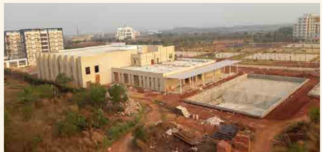
Swimming Pool: Structural work completed. Finishing work is in progress.
