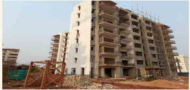
Type-C3 Quarters: Structural work completed and finishing work is in progress.
