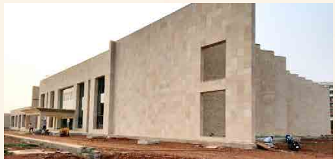
SAC: Finishing work is in progress. About 93 % of building work completed
