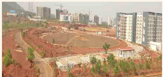
Cricket ground: About 60% work completed.
