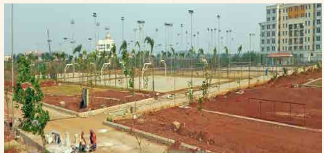
Basket Ball Volley Ball & Tennis Court: About 90% work completed.
