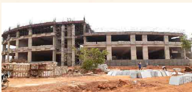
LHC-2: Structural work 70% completed. About 43% of building work completed.
