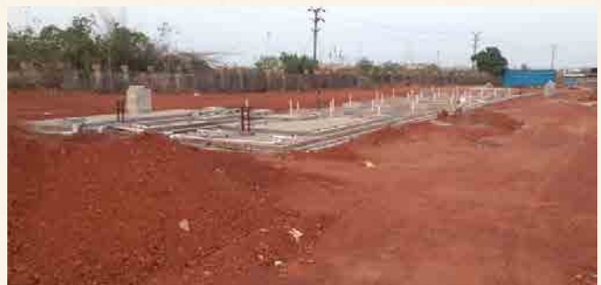
STP: About 90% of STP work completed.
