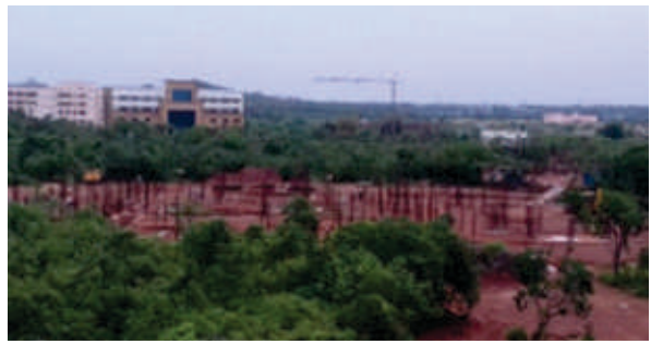
SMMME: Plinth beam and earth filling work is in progress
