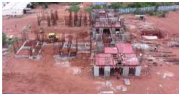
D Type Quarters: Front side roof slab shuttering work is in progress.
