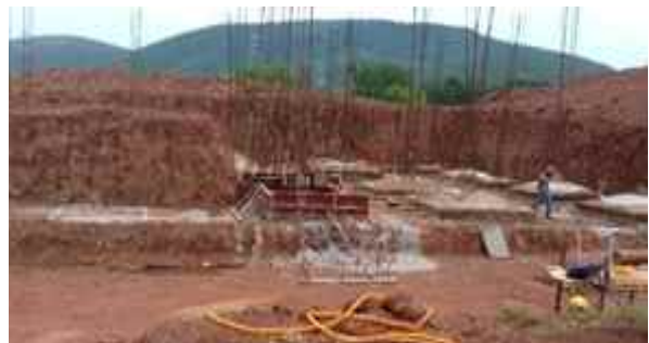
Dispensary: Column footing work is in progress.
