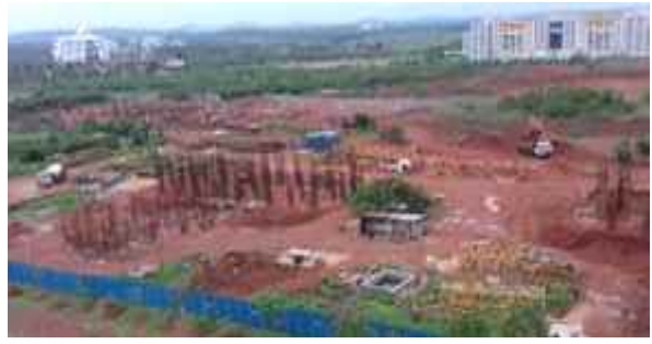
Type-C3 Quarters: Filling work is in progress.
