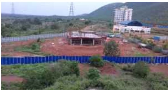
Director's Bungalow: Ground floor slab completed.
