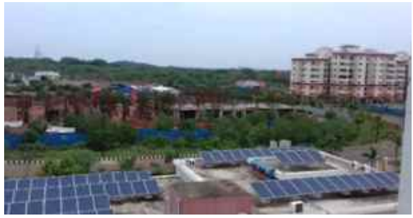
Type-B3 & B4 Quarters: Ground floor slab completed in B4 and B3 column work is in progress.
