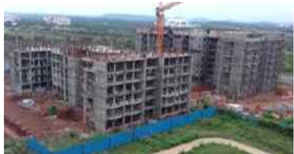
Girls' Hostel- 2: B wing back side 6th floor slab completed& Front side column work in 6th floor slab is in progress.
