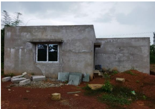
Lab of STP under construction
