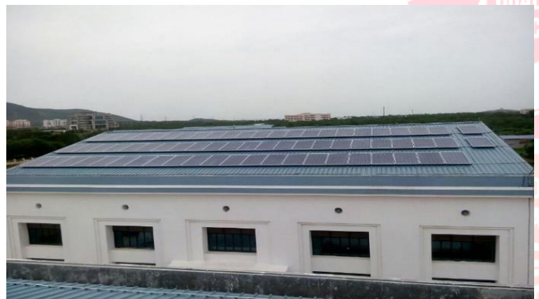
Rooftop Solar PV which was damaged (IIT Bhubaneswar)
