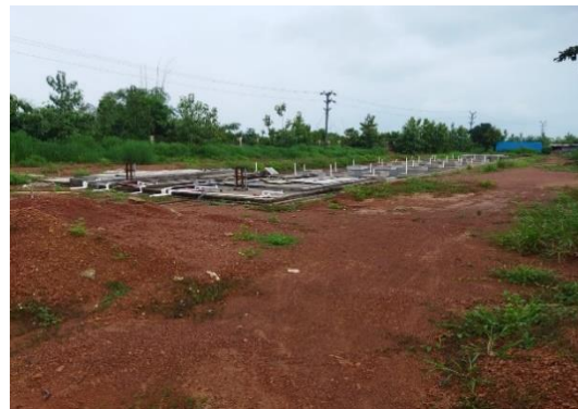
Lab of STP under construction
